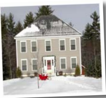
The Maple features a simple frame and foundation.
